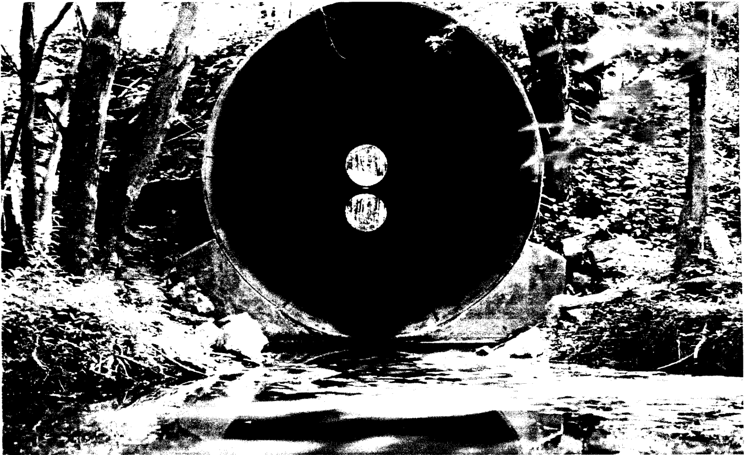
Some portions of the Oxbow are seldom seen by most of the folks visiting Oxbow. This long tunnel, under I-275, Exit #16 road, connects the channels of water behind Mercer Pond to the lake north of the exit #16 road. At high water the flooding Ohio and Great Miami River waters flow through this tunnel to flood the area north of the exit. (photo by Wayne Wauligman)
